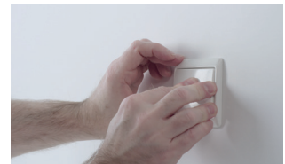
04 Mount the cover of the pushbutton.
